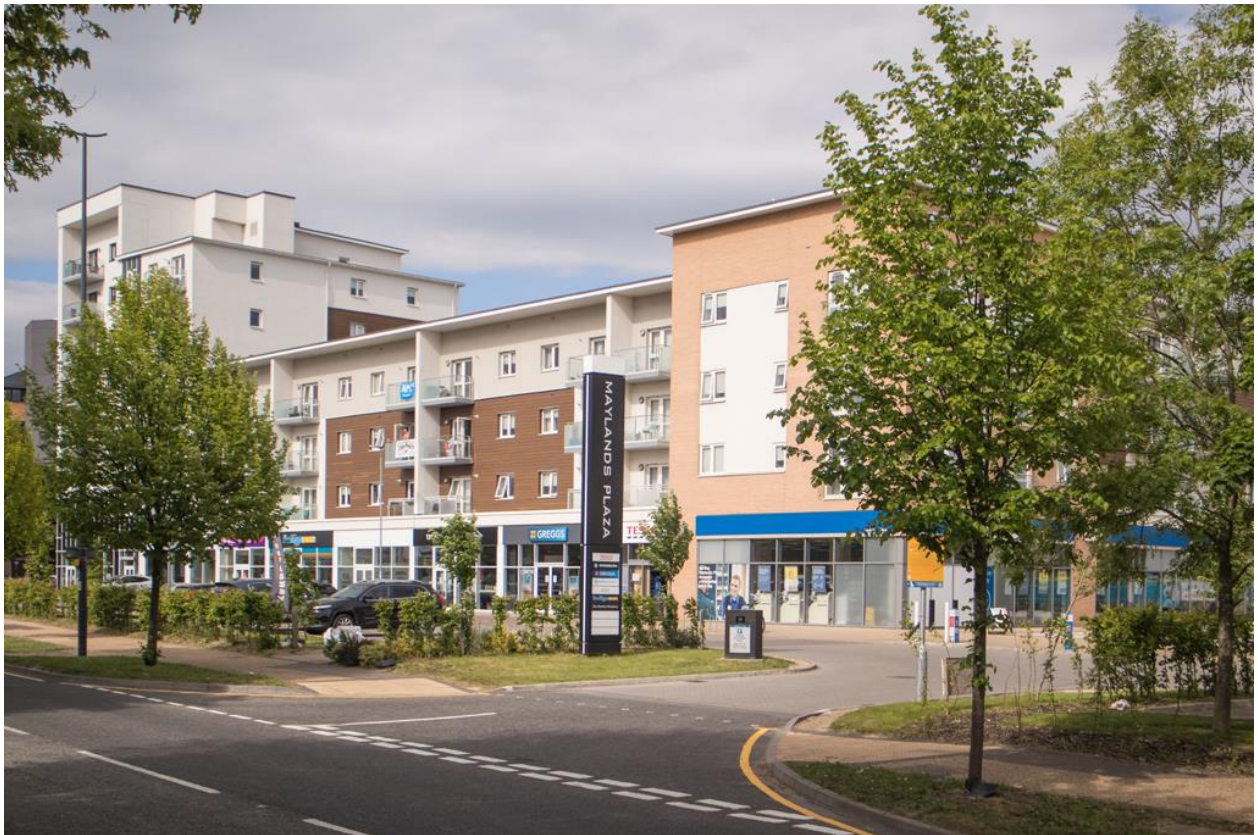
Affordable rented housing at Maylands Plaza, Maylands Avenue, Hemel Hempstead (Hightown Housing Association)
